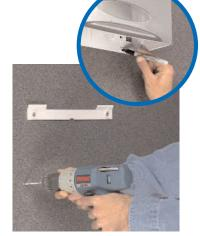
5 While dispenser is hanging on wall bracket, mark bottom two anchor locations. Pre-drill the bottom holes using a #25 drill bit.
