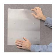
3 Remove second paper covering on each pad to expose adhesive. Reverse wall plate and position it on wall. Make sure the four bolts are protruding and the two closer together are at the top. Press firmly to adhere plate to wall.
