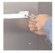
4 Line up the holes in the mounting bracket with the top pair of bolts. Place a nut on each screw and tighten (turning clockwise) to secure bracket on wall plate.
